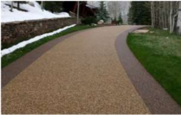
Fig. 8: Application of permeable concretes
