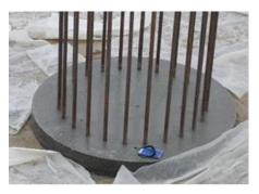
Fig. 19 Pile Head Waterproofing System
