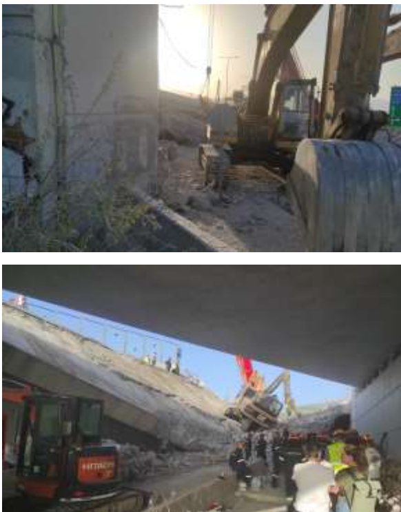
Figure 2. Collapse due to uncontrolled demolition of a bridge at the North entrance to Patras (Greece) collapsed on 2023/7/23 (Author's photographs).
