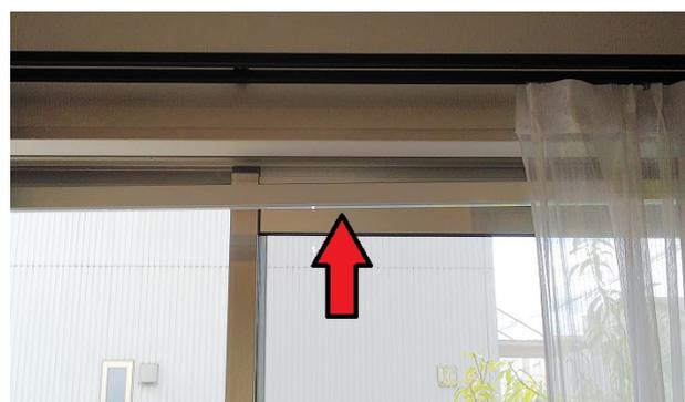
**Figure 8:** The SAWOACSS device from Sanko Co., Ltd., installed to automatically open and close windows. The arrow points to the SAWOACSS, mounted at the top of the window.
