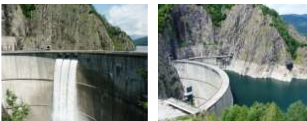
Fig. 2: Front and side view of Vidraru Dam and hydropower plant Vidraru
