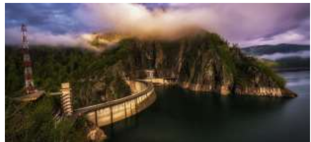
Fig. 1: Top view of Vidraru Dam
